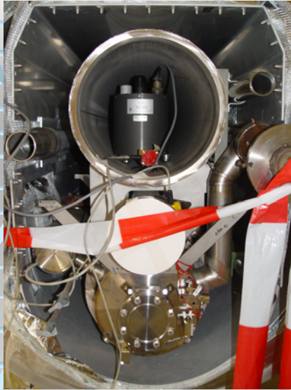
Seismometer Güralp CMG-6TD inside Helium Gas Return Pipe (GRP)
