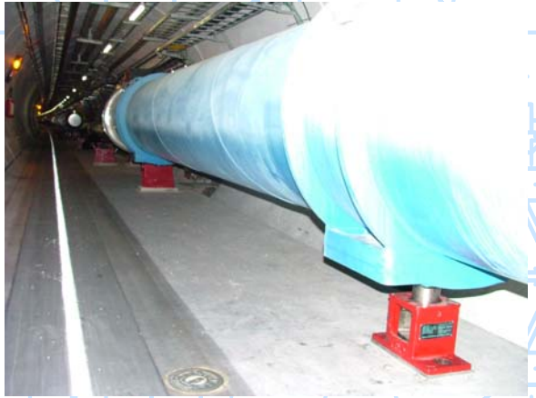
LHC standard cryodipole installed in the 3-4 arc section
