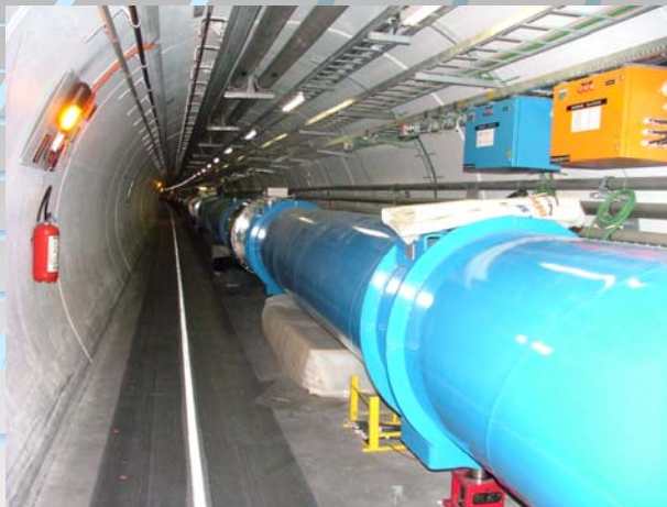
LHC tunnel, CERN
