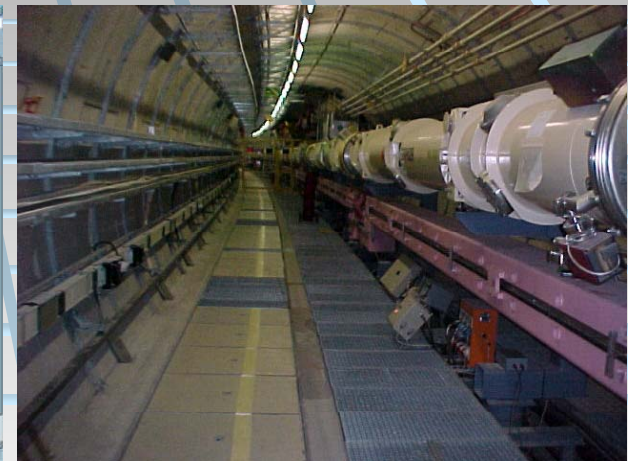
HERA tunnel, DESY
