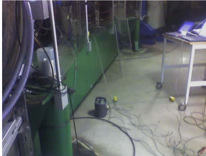
Figure 2: Measurement of the floor vibration near the girder with the seismometer and simultaneously, with both vertical and horizontal geophones
