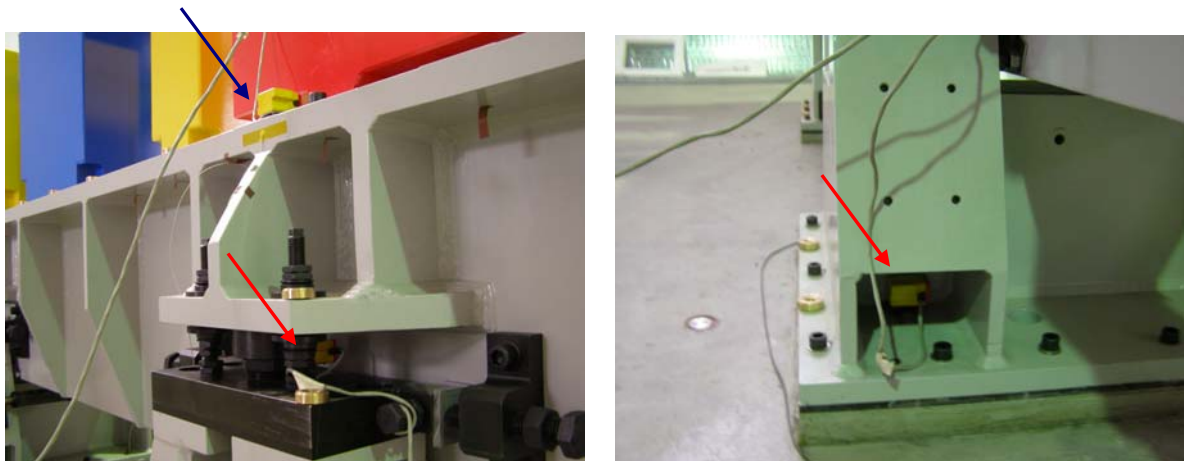
Figure 3: Positions of geophones to measure transfer function in going from the girder top (blue arrow left) to the pedestal (red arrow left) and the pedestal base plate (red arrow, right).
